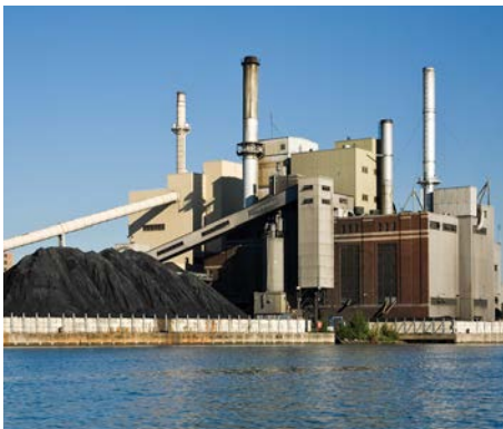
Metal expansion joints are installed in flue gas piping systems.
