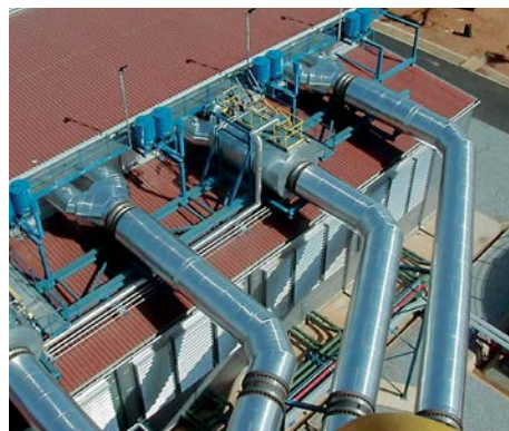
US-type flue gas metal expansion joints are designed for positioning in the flue exhaust gas system.
