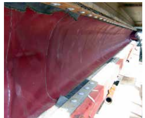
Fluachem Fluoropolymer installed in a vertical duct.
