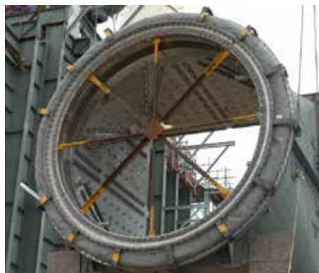
Installation of Combine-X on diffuser.
